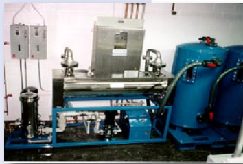
After UV installation
