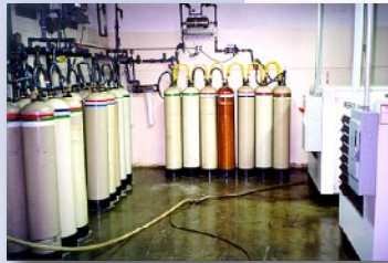
Before UV installation
